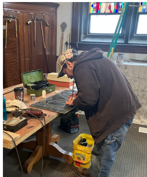
Repairing Stained Glass on Site
