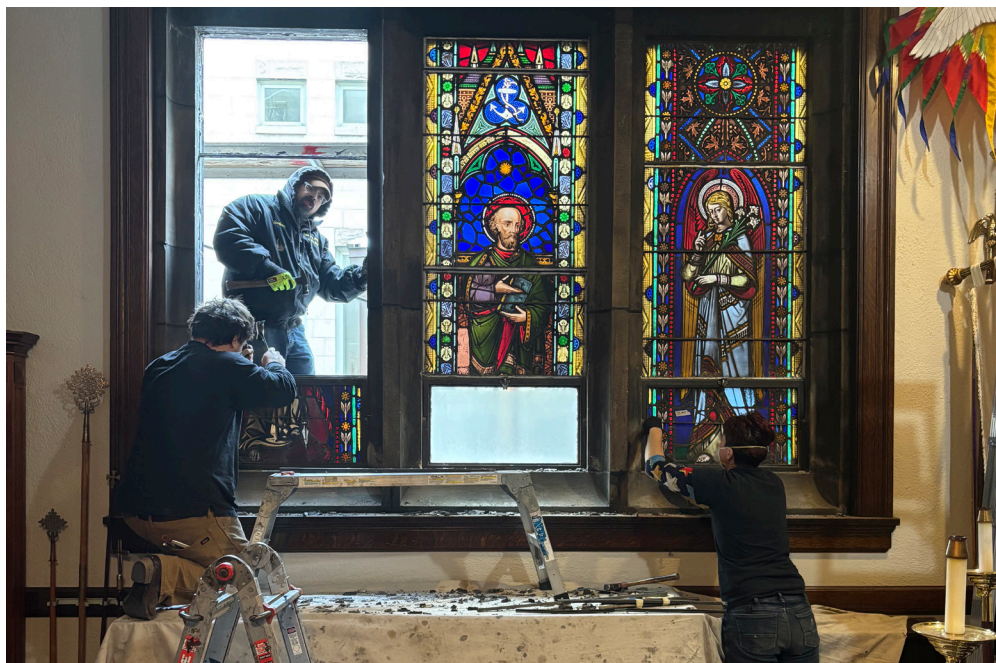
Replacing Stained Glass in Vesting Room
