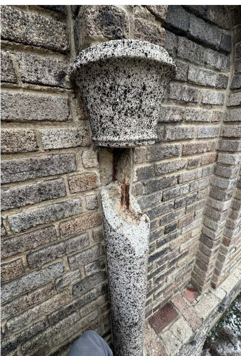
Repairs to Exterior Stone Work
